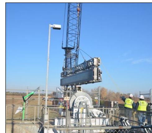
Steel bulkheads are lowered into the water to shut off the spillway so engineers can open and close the dam gates, Nov. 5. Photo by Elizabeth Stoeckmann
